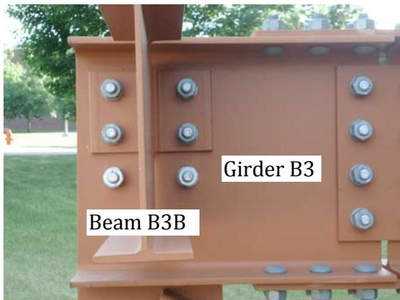
**View C. Double bolted-welded-angle shear connection, back of View B**
