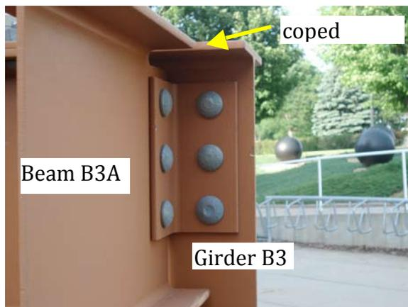
**View A. Double bolted-angle shear connection**
